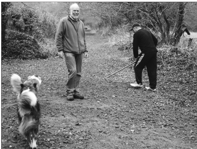
Laying new scalplings on the Dram Road where the path was washed away by excess surface water Gosod cerrig mân ar y Dram Road lle golchwyd y llwybr i ffwrdd gan lifogydd
