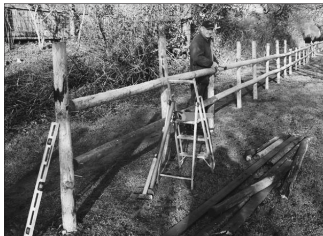
Replacing rotten handrails Ail-osod canllawiau powdr
