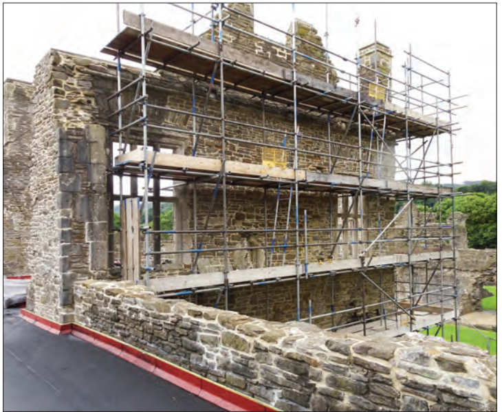
Re-pointing the Tudor house
